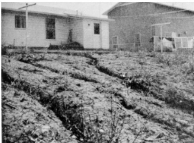
Figure 33.—Erosion in ungraded yards.
