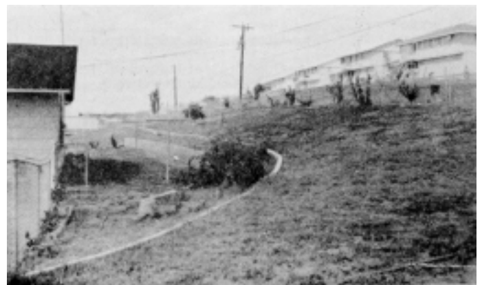
Figure 34.—Terraces and retaining walls built to prevent water erosion in landscaped yards.
