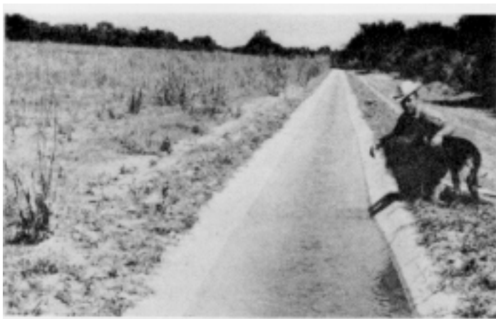
Figure 20.—Concrete-lined ditch. The lining will prevent loss of water.
